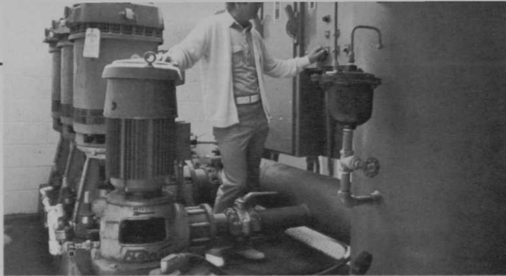
The pumping plant is the heart of the system. Superintendent Sonny Faust had this one installed when modernizing his irrigation system at Southern Hills CC in Tulsa.
