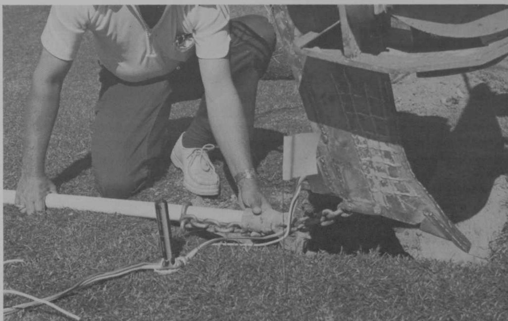
Pipe is attached to vibratory plow blade with pulling grip.
