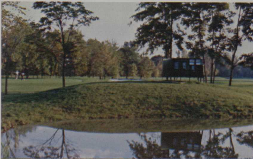
◆ This mound was built out of the floodplain to house pump controls and irrigation clocks.
