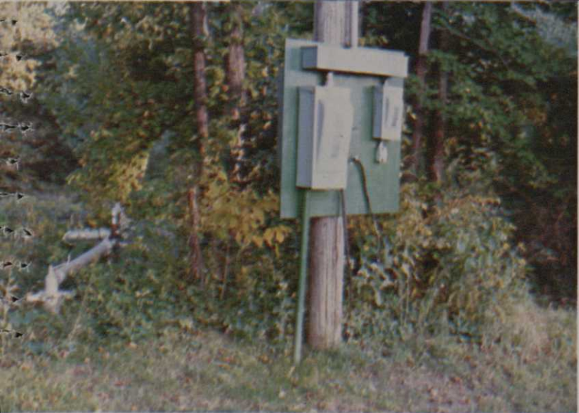
◆ This mound was built out of the floodplain to house pump controls and irrigation clocks.
