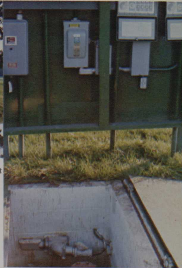
◆ Below is the pit with electrical connection to submersible pump and clayton and isolation valves. Also shown are the pump controls and irrigation clocks.
