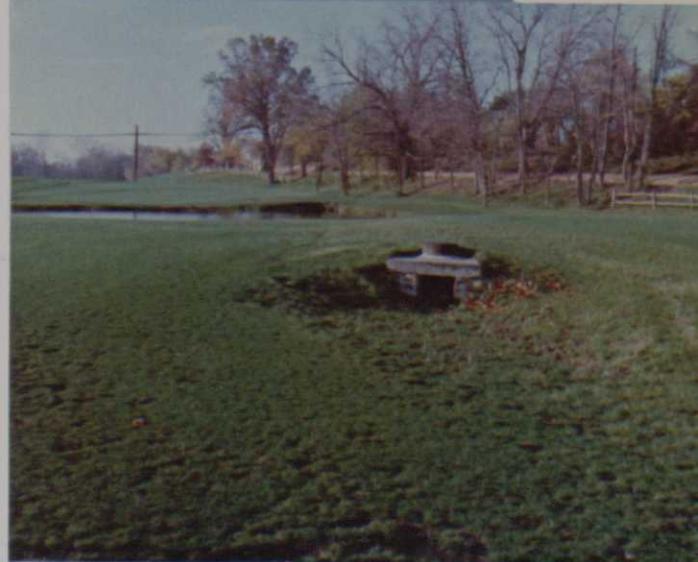
◆ Surface water directed by a grass waterway will flow into this side-opening catch basin.
