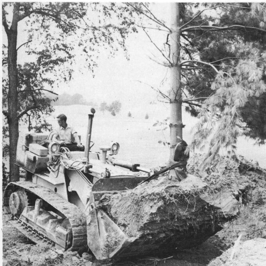
Taking advantage of nature: During construction of the Bellville Project, repositioning of existing trees helped give the course an established look. At the same time, the owners acquired a substantial savings over the cost of replacement stock. Several hundred white pines were transplanted.
