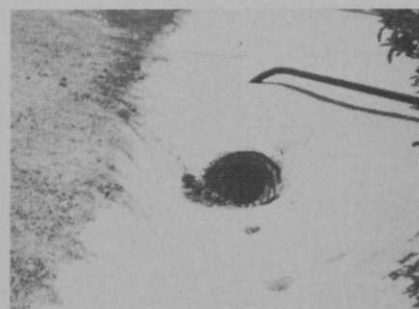
Reject concrete pipe was used on some holes to carry water under the fairways from canyons above so the course would not have water problems on the fairways.
