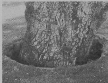
Before work on the course began, every tree was marked six feet from its natural ground level. After grading was complete, every tree was remeasured and if the ground was above the six-foot base, a tree well was built to protect the crown area.
