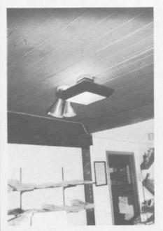
Double lighting effect is an important ploy in highlighting. Spotlights and downlighting fixtures are used to achieve this effect.
