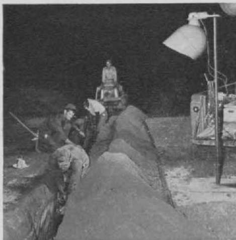
Construction crews worked nights to install a watering system on the 18-hole Broadwater Beach Hotel & GC in Biloxi, Miss. Practically all the work was done between dusk and dawn so as not to disrupt play. Entire project, including the digging of two 1,040-foot wells, was completed in 36 days.
