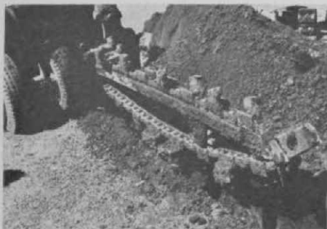
Digging mechanism on the power digger.
