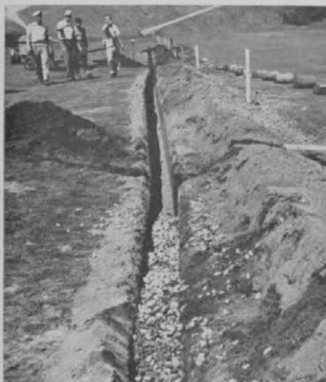
Gravel blanket on top of sand in foreground, and basal sand cover in distance. Note lateral tile line in middle of photo.
