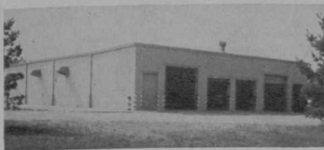
Before and after views of service buildings
