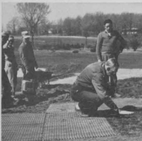
Lyons' planting method avoids objectionable foot-printing on planted areas. One of the steel mats supports the man who scatters the stolons.
