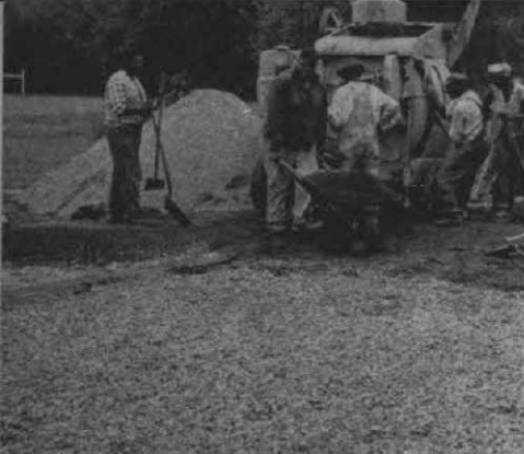
Danner supervised building of three bent greens at Belle Meade, also in Nashville. In foreground is gravel sub base; at rear topsoil is being mixed.
