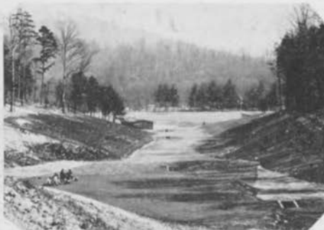
A view of the 10th fairway, showing four of the special inlets.
