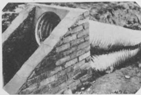
One of the special inlets during construction. The sloping face is later screened over.
