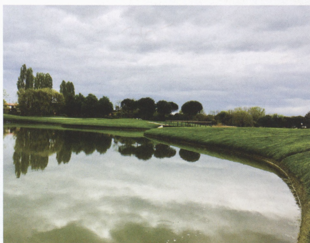
Lignano Golf Club rebuilt lake edges using the AquaEdge method. The project was split in two solutions based on the depth of the standard level of water near the edge.
