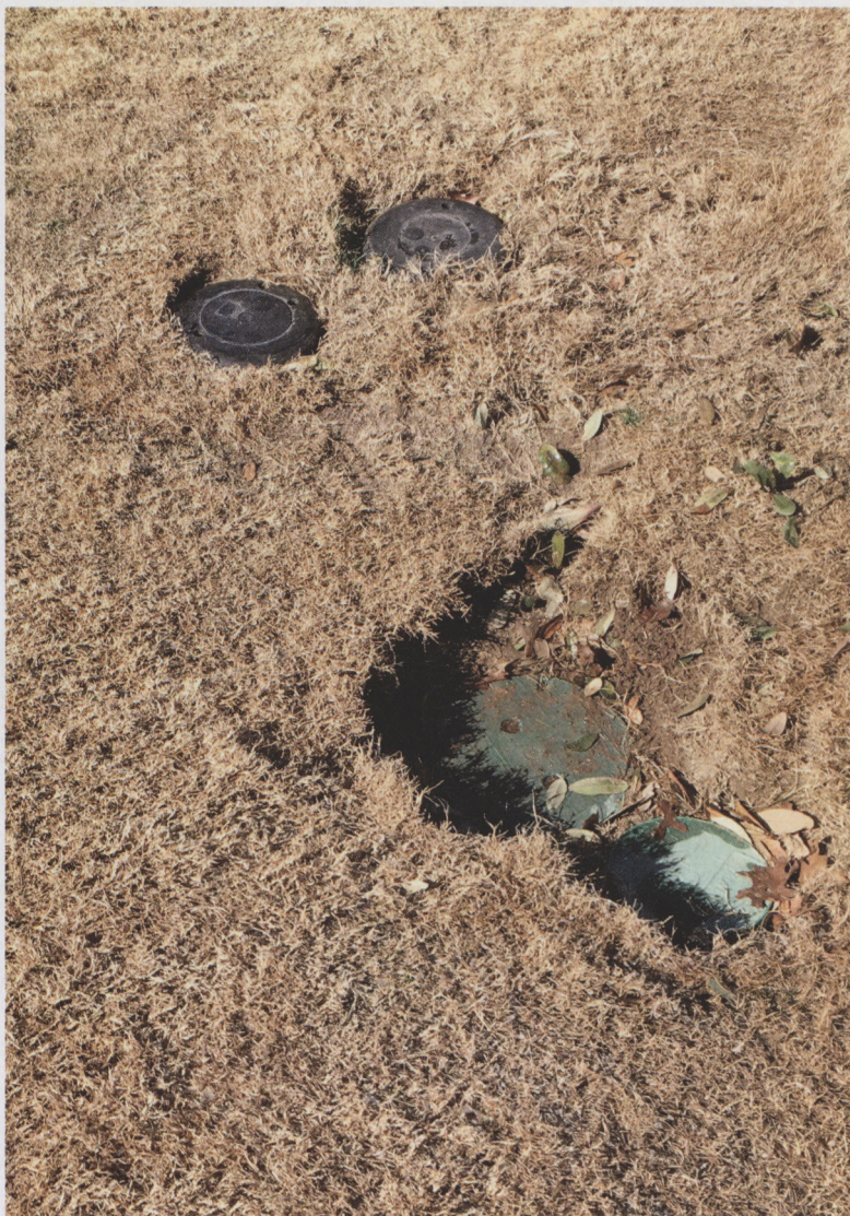
Below-grade components of an irrigation system can create risk management issues for a golf course.
