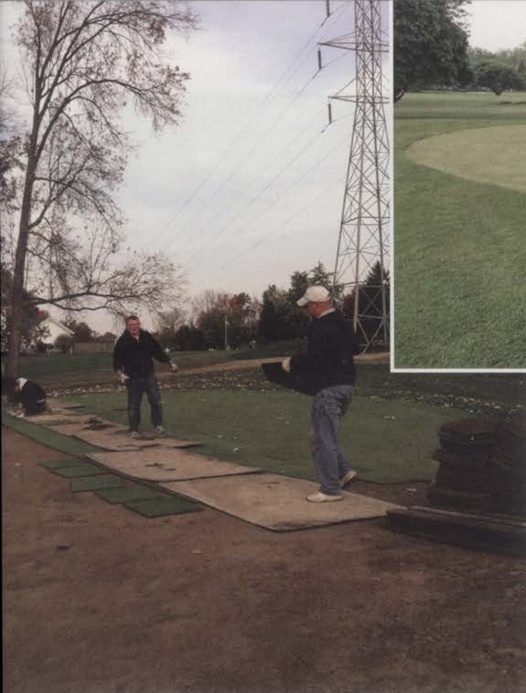
Recapturing lost green space as part of a greens reconstruction can help disperse foot traffic and increase pin locations on the putting surface while expediting the movement of water out of the profile.
