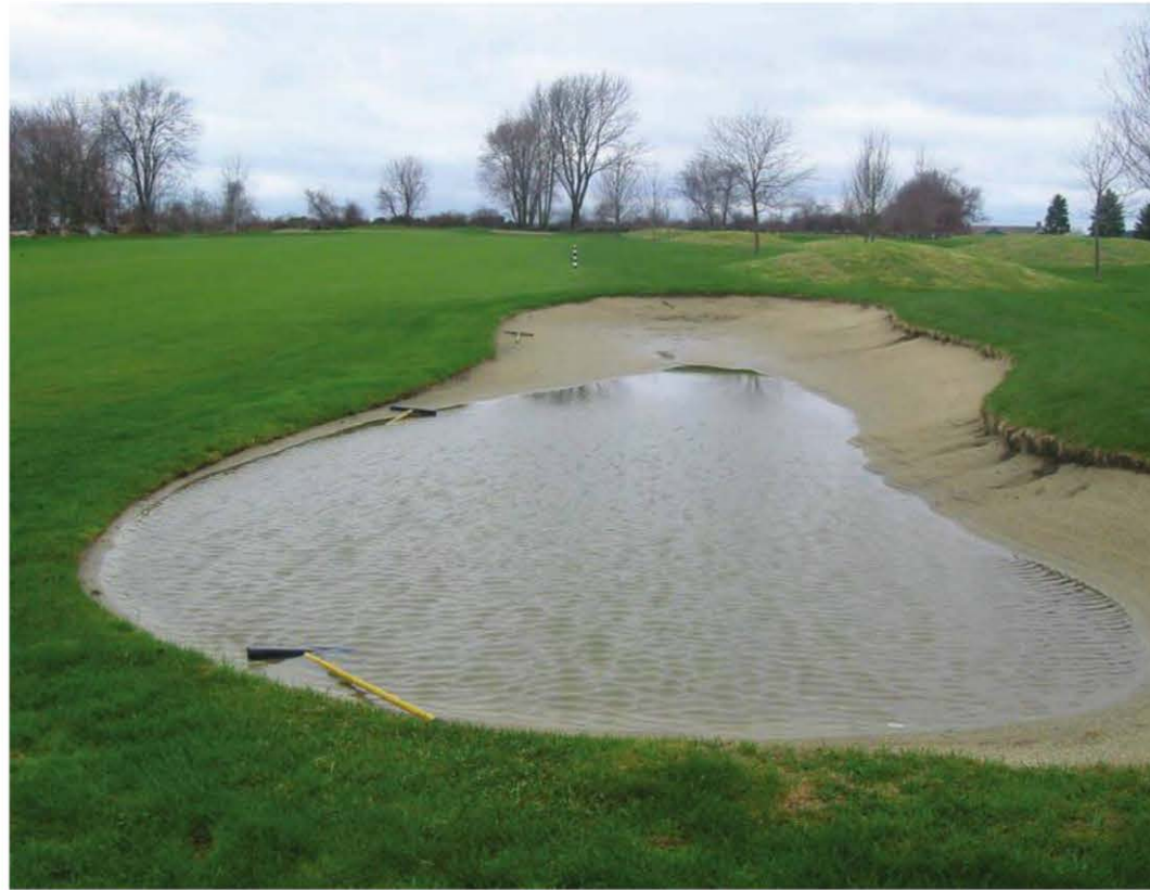
Bunkers without proper drainage create major problems and require hours of additional maintenance for superintendents and their crews.
