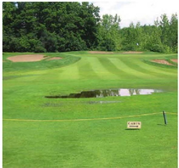
Ponding is a common fairway drainage problem that disrupts cart traffic and slows place of play.
