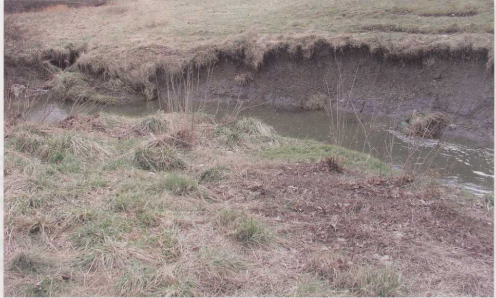
The 14th hole at Lost Nation Golf Course in Willoughby, Ohio, before the completion of a major stream restoration project. Ward Creek, which flows through the back nine, was experiencing severe erosion, leading to sediment runoff entering the Chagrin River. The river flows into nearby Lake Erie.
