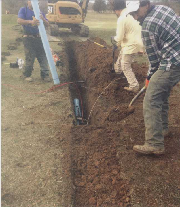
Time-consuming and expensive repairs led to Port Jefferson Country Club on Long Island replacing its irrigation system. Renovations at the club also included a bunker restoration project. The course reopened this past spring.
