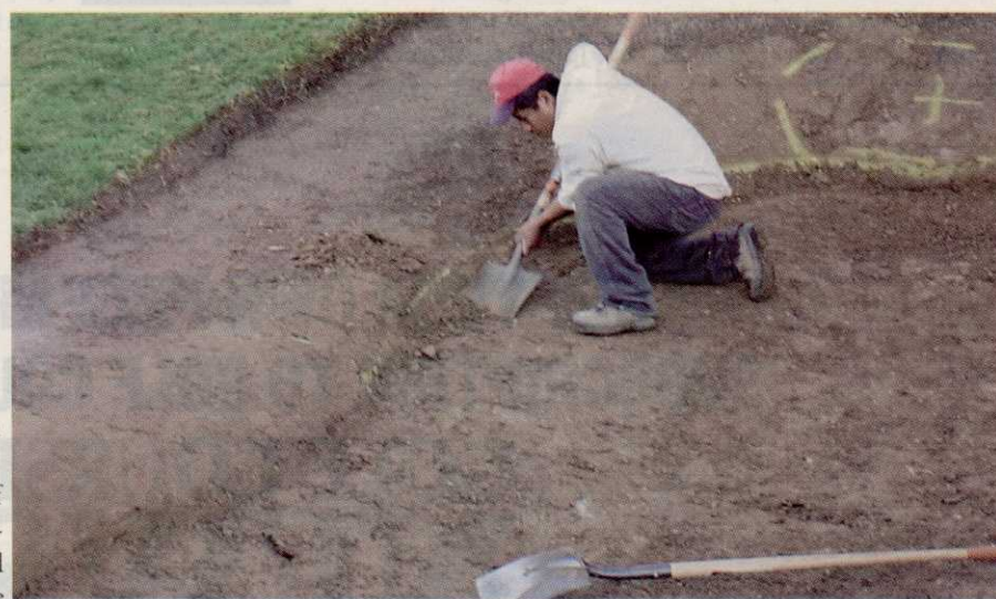
A worker excavates a bunker to bring back the fat lip of Fazio's original design.
