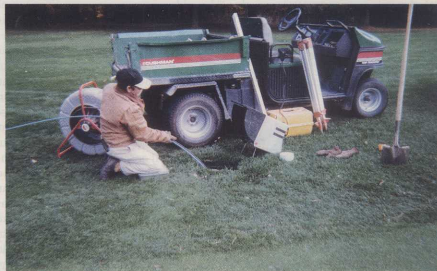
A worker feeds the See Snake into a drain to scan for any blockages or crushed tiles.
