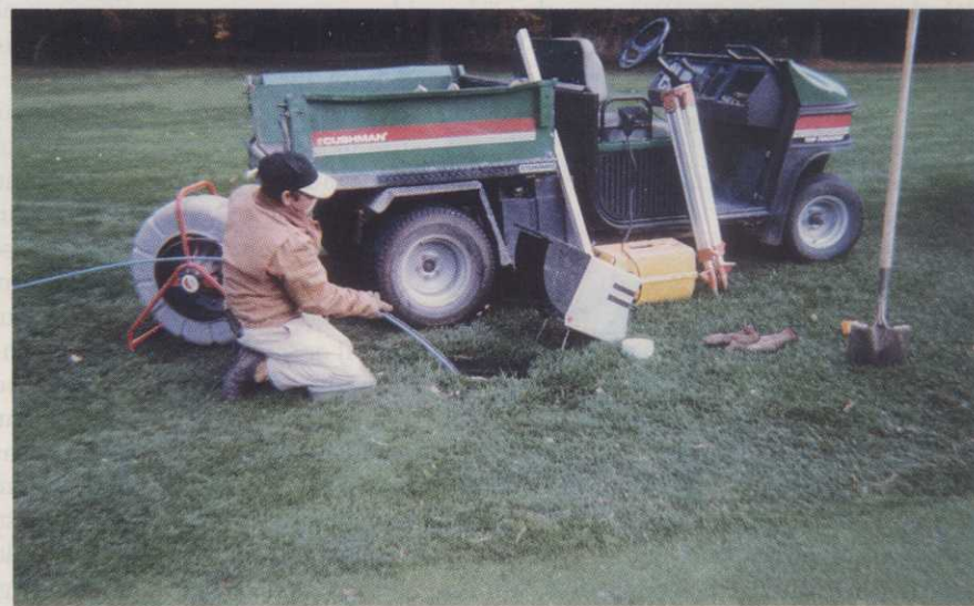
A worker feeds the See Snake into a drain to scan for any blockages or crushed tiles.
