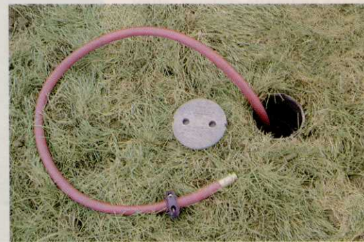
The pressurized, retractable hose is hidden underground.
