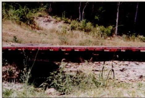
The bridges at Buck's Point GC were constructed from the decks of old tractor-trailers.
