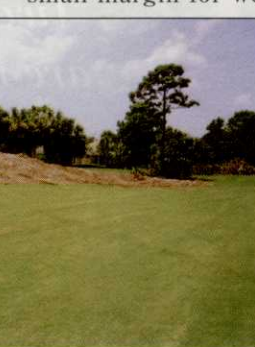
Creation of a more visible fairway bunker complex on the 17th hole was completed by generating all of the necessary fill from on-site.
