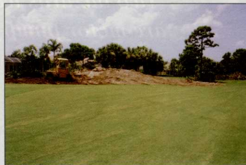
Creation of a more visible fairway bunker complex on the 17th hole was completed by generating all of the necessary fill from on-site.
