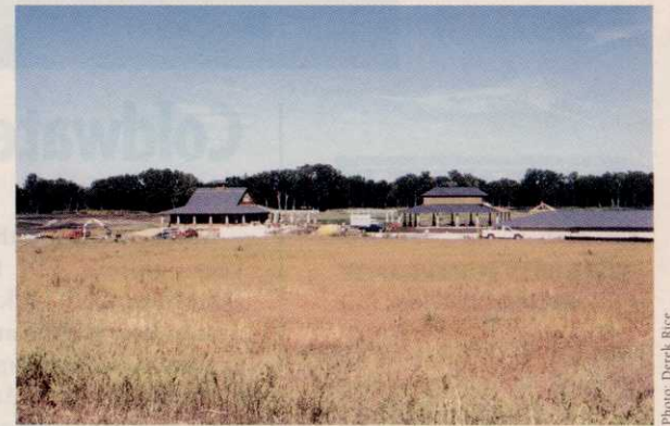
Construction continues on the clubhouse at Coldwater Golf Links.
