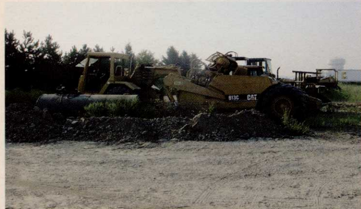
Construction equipment sits idle at the site of the planned Desert Challenge.
