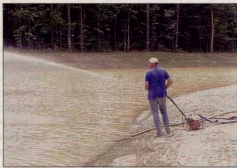
Gypsum being dispersed with a hydroseeder
