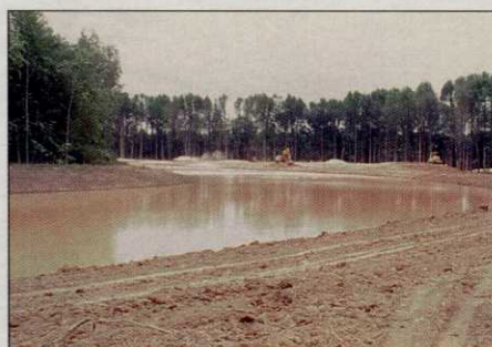
Patriots Glen's irrigation pond before...
