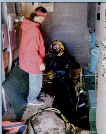
A diver from AUS entering a wet well
