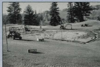
Approach renovation with sand rootzone, extensive drainage, and independent irrigation may become the standard.
