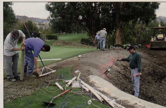
Renovation work is underway at Silver Creek
