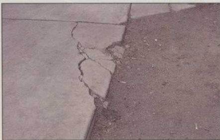
Golf car paths need to be free of trip hazards
