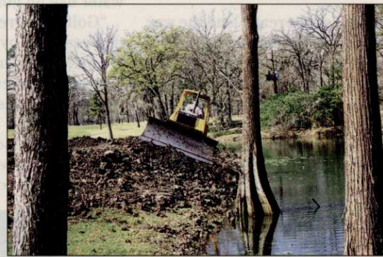
A bulldozer builds up a green slope at Houston's Lakeside Country Club.
