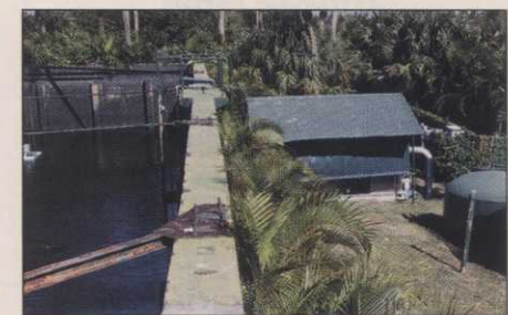
A storage tank keeps a ready supply of effluent.
