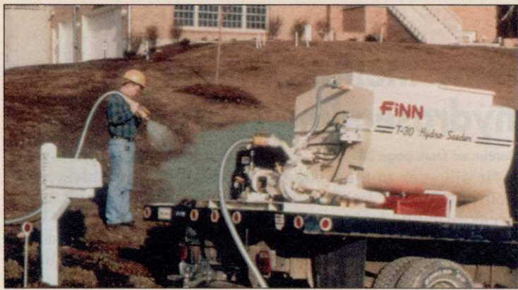
Laying down the Finn Additive System.
