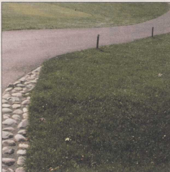
Plain, inexpensive stone curbing serves the purpose of saving pathside turf.
