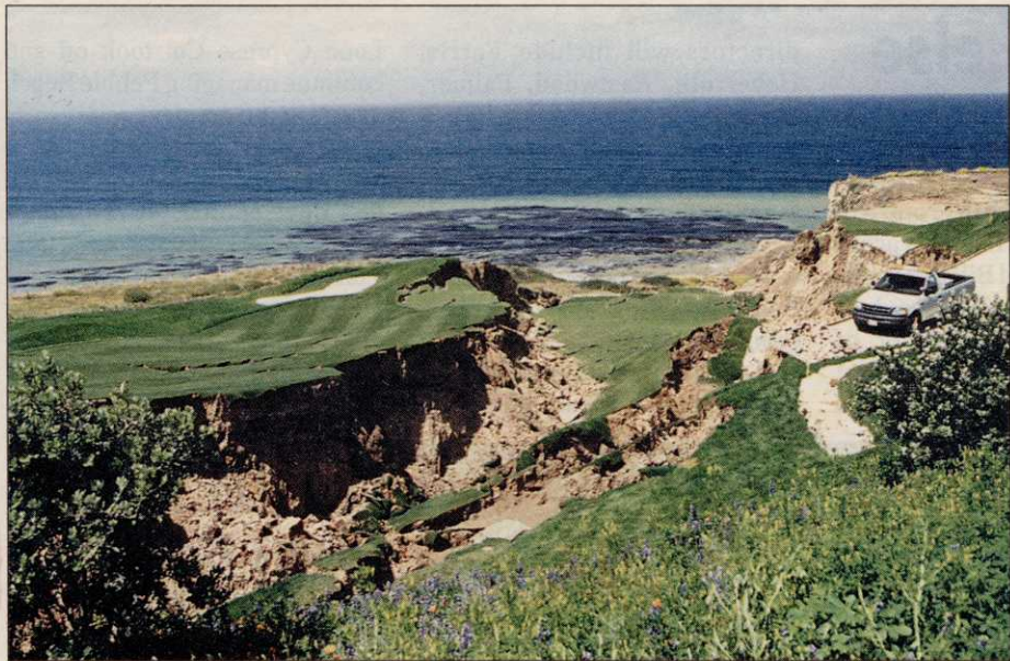
Developers of Ocean Trails Golf Course in Rancho Palos Verdes, Calif., are still seeking a solution to repair the landslide that pushed part of the 18th hole toward the ocean in early June.
