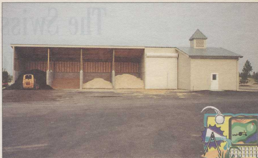
The five-bay combination soil-/fertilizer-storage building at Cottonwoods Golf Club.
