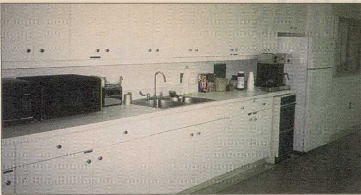
Modern, efficient golf course turf-care centers provide a state-of-the-art kitchen facility in the employees' lunchroom.
