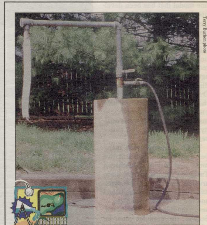
Filling a truckster-mounted or towable sprayer with water is easier with this simple devise.
