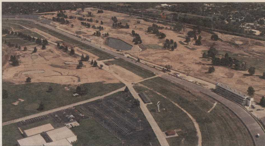
The newly renovated Speedway course will feature 18 holes — down from 27 — with four inside the oval.
