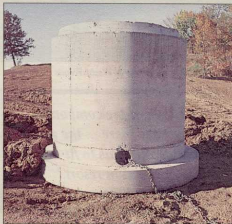
Basins like this have been installed at each hole at the Outlaw Course. Note the inflow hole at the top of the basin and outflow hole on the bottom of the other side. This allows a gravity flow over filtration material before the water leaves the site.
