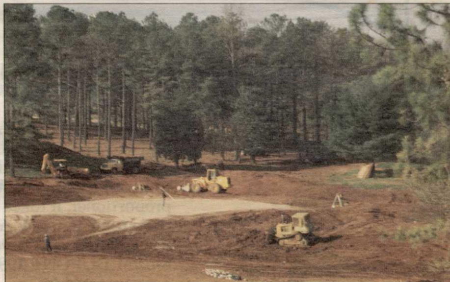
To better accommodate increased traffic, the first green at Marietta Municipal GC is being rebuilt.
