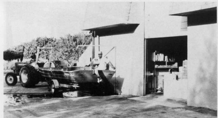
Boca Greens chemical room is designed with easy entry, concave floor with drain, sink, and outside hose bib. ■
