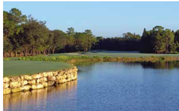
Stacked capstone replaced timber retaining walls and reinstated the levels between putting surfaces, collars and hazards.
