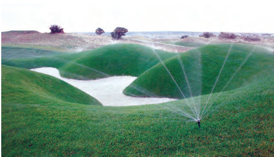
With multi-stream, multi-trajectory rotating technology, the MP Rotator (shown here) delivers water at one third the rate of spray heads which allows the tight soil on bunker faces to efficiently absorb the water it needs--producing a healthy, green stand of turf. This technology has gradually started to infiltrate the Florida market.
