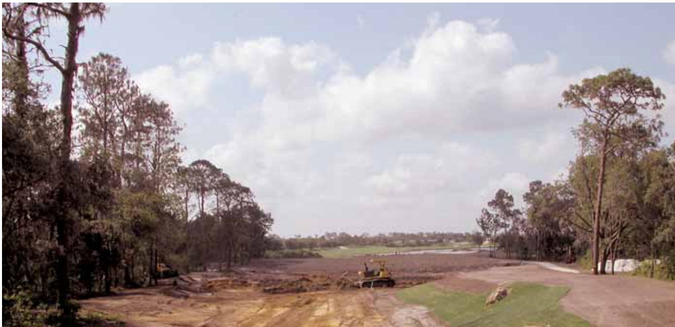
A large stormwater retention area is part of the redesign of the 17th hole. The tee tops and fairways have been sprigged and erosion-prone areas are being sodded. Photo by Joel Jackson.
