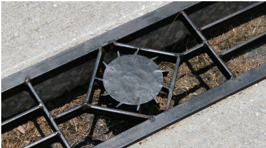
This decorative grate across this cart path was created from an old mower reel by Equipment Manager Larry Jordan. Several paths were cut to provide drainage for water trapped on the course. Photo by Joel Jackson.
