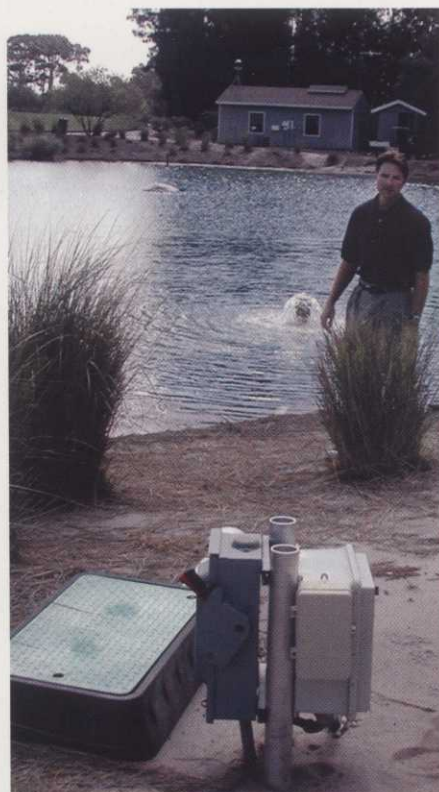
Tom Trammell, CGCS, stands in front of the horizontal well installed more than one year ago. The well provides more than 300,000 gallons of water per day for irrigation usage. Trammell notes that he has made sizeable savings over the last year due to improved water quality and reduced electrical cost for pumping from the shallow source. Hawk's Nest is scheduled to add one more well in the summer of 2002.
